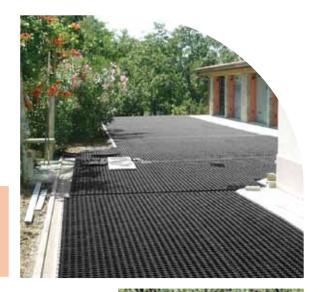
Permanent grassed or gravel car parks, fire access routes, cycle paths, driveways, access roads and other trafficked areas where a structurally-sound, well drained base is present or will be installed.
