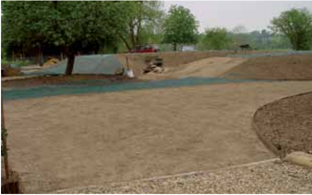
Newly landscaped installation using green TURFPROTECTA laid and covered with a layer of topsoil and seed.
