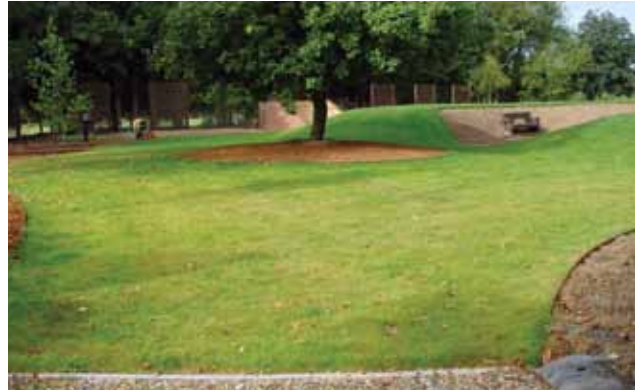
After just a few weeks the grass grows through the mesh offering a strong stabilised surface.
