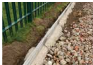
Edging kerbs installed
