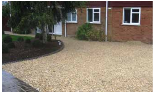
Filled with angular gravel creating an attractive reinforced permeable surface that retains the gravel
